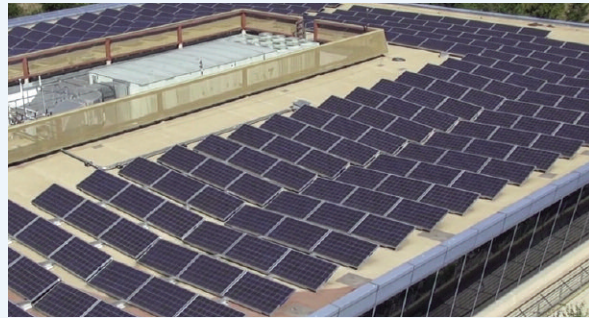
Figure 4 - Solar Panel Inspection
